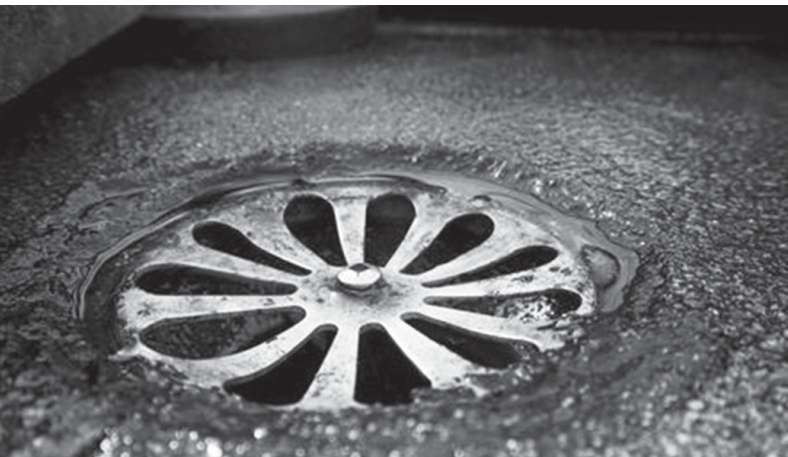
A drainage system that led to a floor drain in another room, built by a janitor to deal with a leaky boiler, was only a temporary fix. A much bigger problem loomed.
